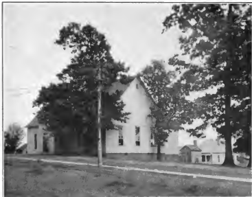
PUBLIC SCHOOL BUILDING, DRAKESBORO
